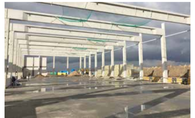
» On stage of the construction
